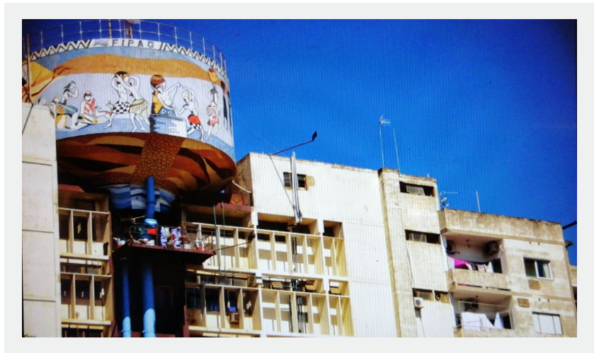
Image 12: Example of integrated water tanks in buildings (in the cement city and urban periphery). Source: CRPP 2019.
