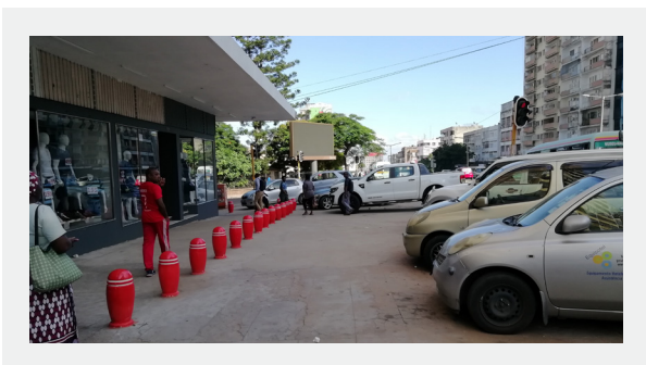
Image 22: Physical elements, allowing the “coexistence” between pedestrians and cars. Source: CRPP (2019).
