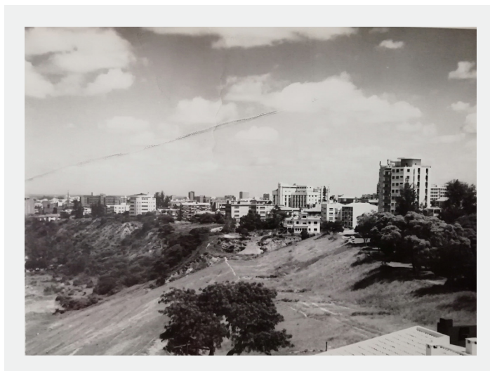
Image 14: Earthworks for the construction of the descent road to Baix.
