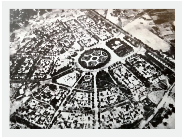
Image 1: Aerial view of Munhuana's neighbourhood.
